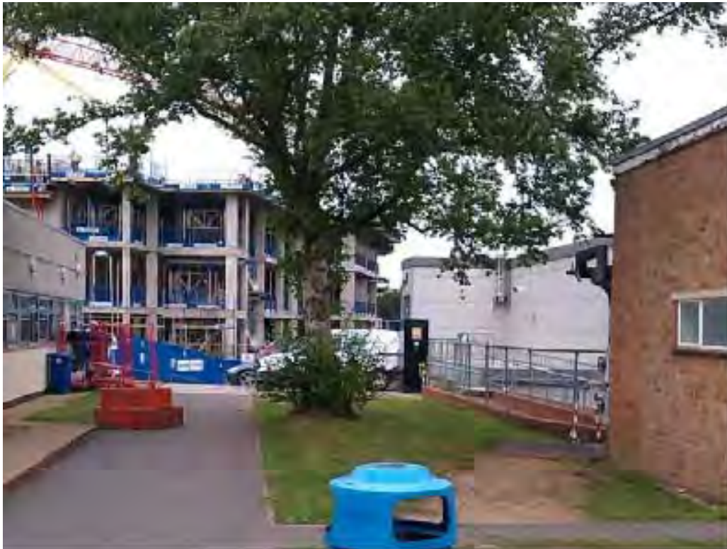
View from OPD/X Ray Corridor towards phase 2a building
